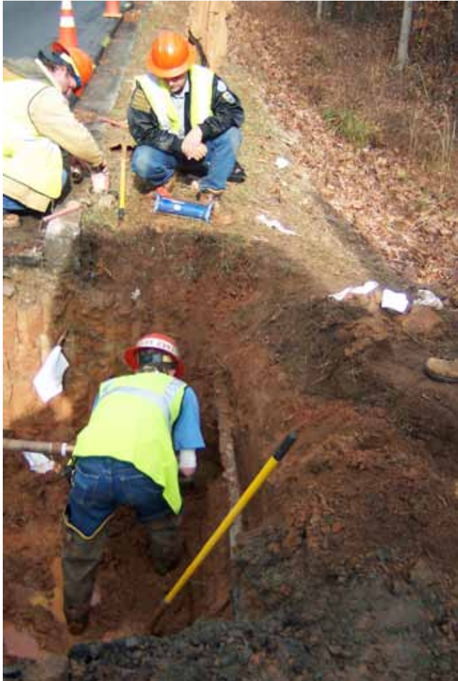
The Cobb County (Ga.) Water System took several actions after losing 8% of its work force. One program created an internal training and certification program in such areas as excavation and trenching.
